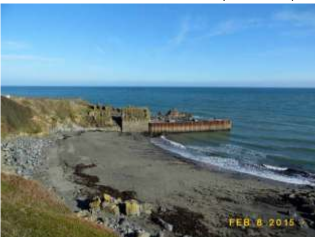
Figure 40: The existing jetty
