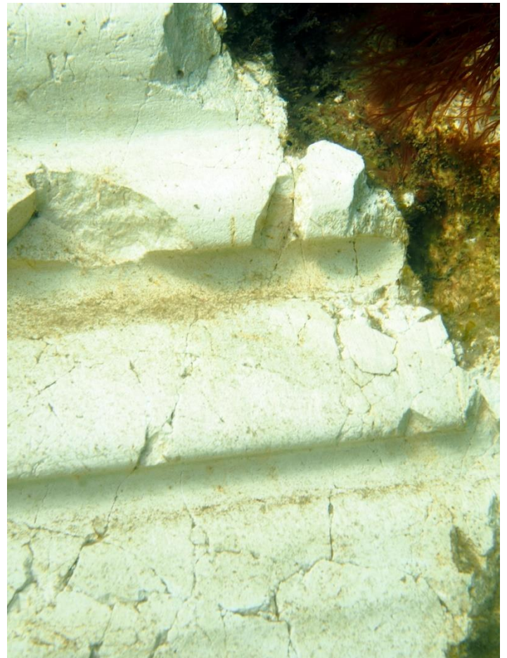
Typical rope cut damage – the position of the rope is reset on every tide
